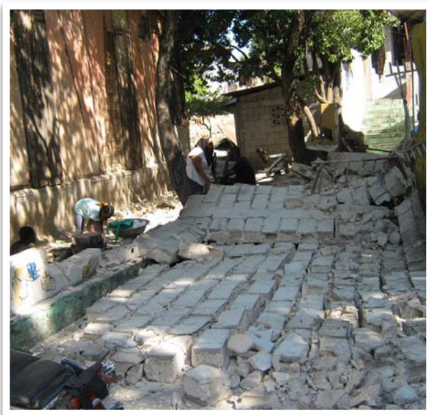
One of the walls that surround the school collapsed. Fortunately no one was hurt. Ours was one of the few schools in Port au Prince not to suffer extensive damage. Many were entirely destroyed.
